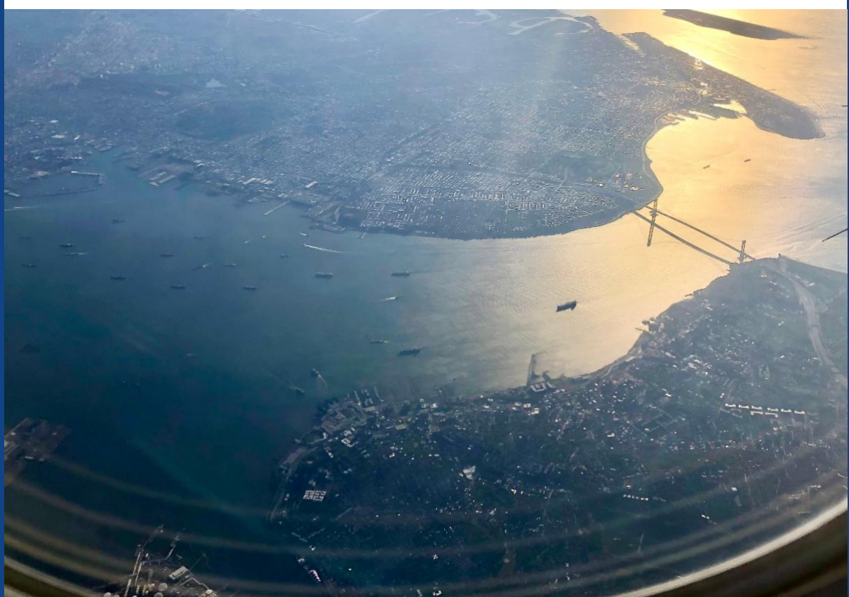
Top: The Verrazzano-Narrows Bridge looking toward Staten Island
