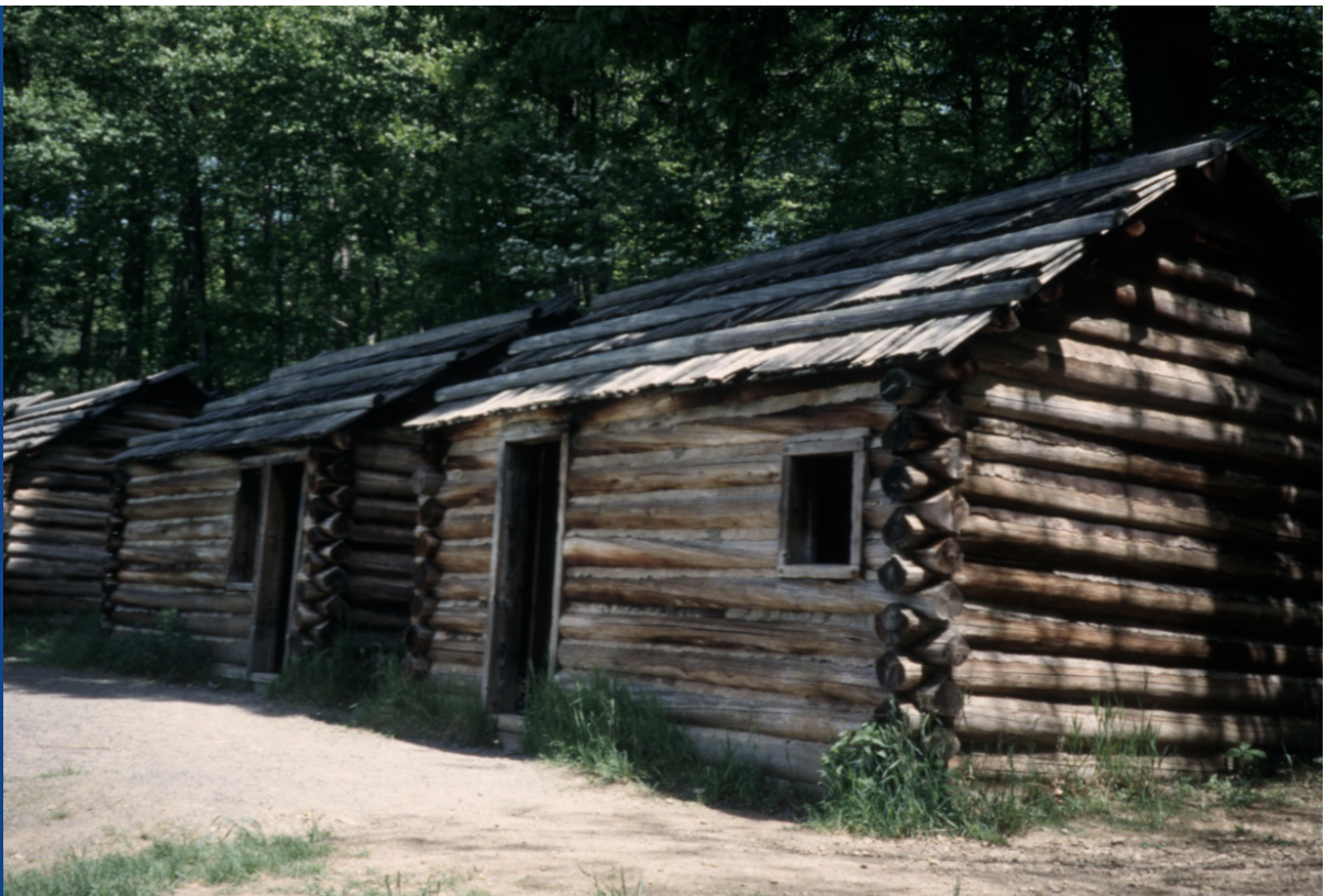
Fig. 2. Soldier huts. The soldiers built two thousand huts similar to these to house 20,000 men and officers. Each hut sheltered nine to twelve men. Construction was completed in a month, and the encampment became the fourth-largest city in America after Philadelphia, New York, and Boston.
